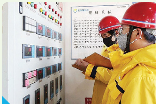
Gas transmission pressure is monitored
