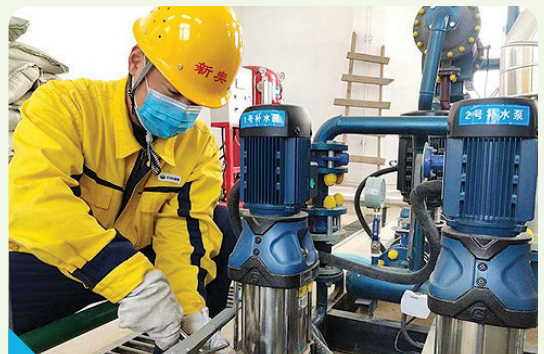
A Shijiazhuang ENN employee is maintaining the pipeline
