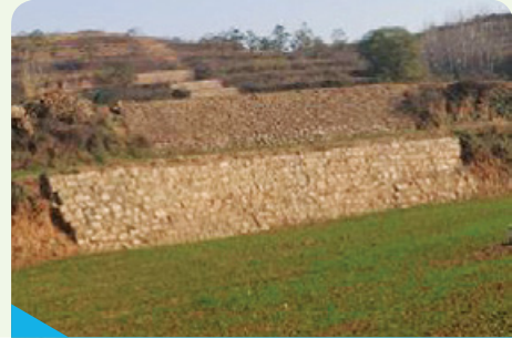
A cofferdam was built to keep water and soil
