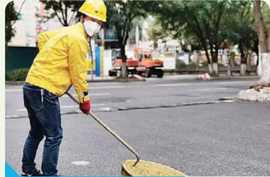
A staff member inspects a valve well
