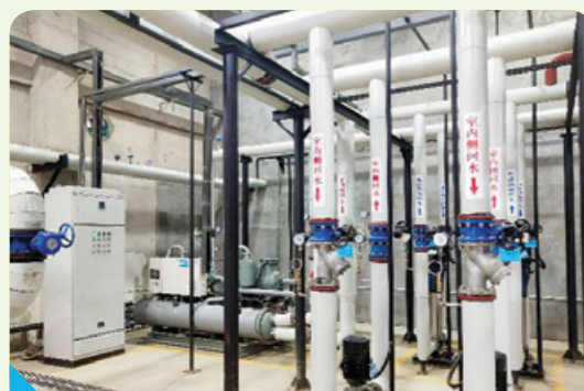
Workshop of our innovative geothermal heating solution
