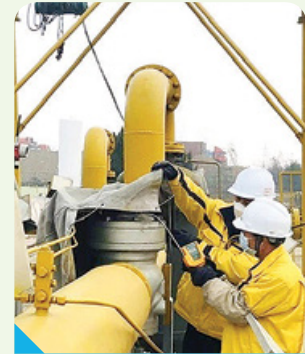
Leakage detection of the high-pressure pipeline at the Menci Station
